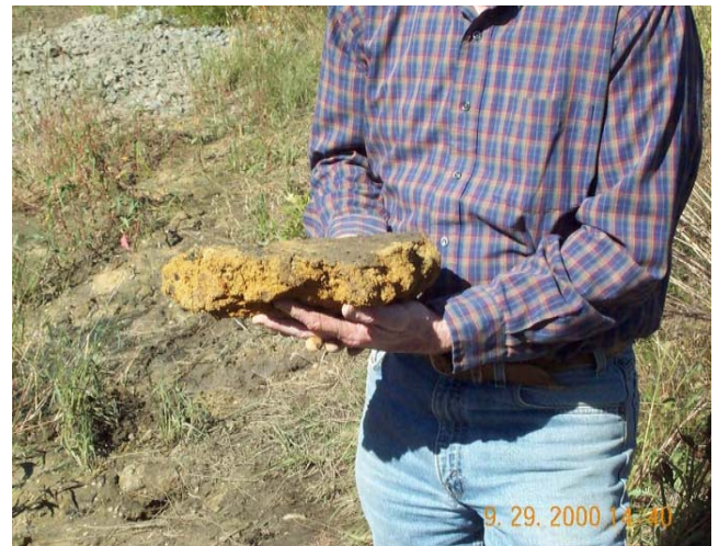
Compacted subsurface layer causing stormwater basin not to function due to lack of infiltration.
